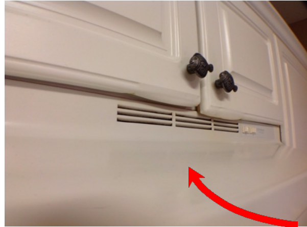
Upper Cabinets - Cabinets door swelling.
